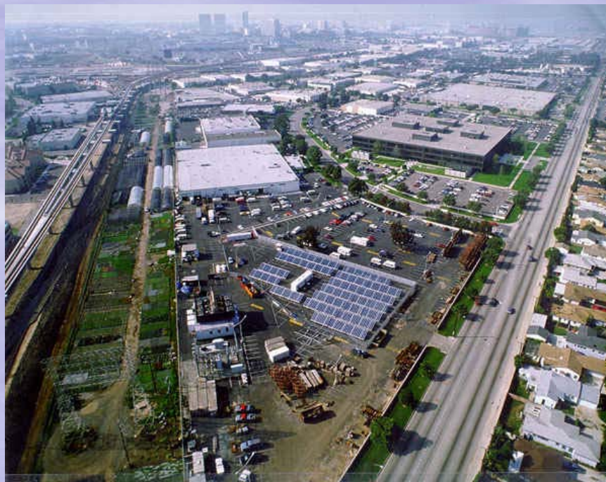
DOE-funded facility for hydrogen-fueled vehicles and fuel cell buses located at Xerox Corporation in El Segundo, CA
