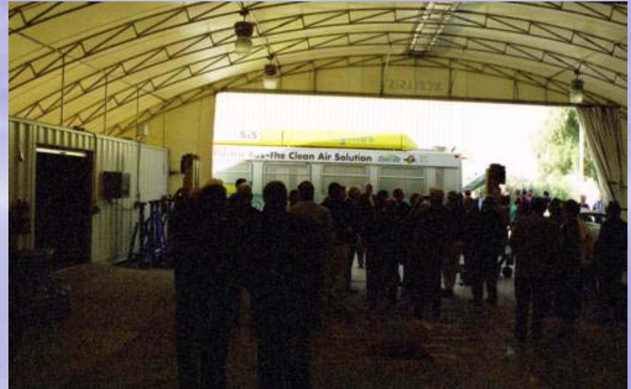
SunLine service building. The structural frame is covered with cloth. A vent runs along the length of the roof making it impossible for any escaping hydrogen to be trapped. Local codes recognizes this building as essentially an “outside area”
